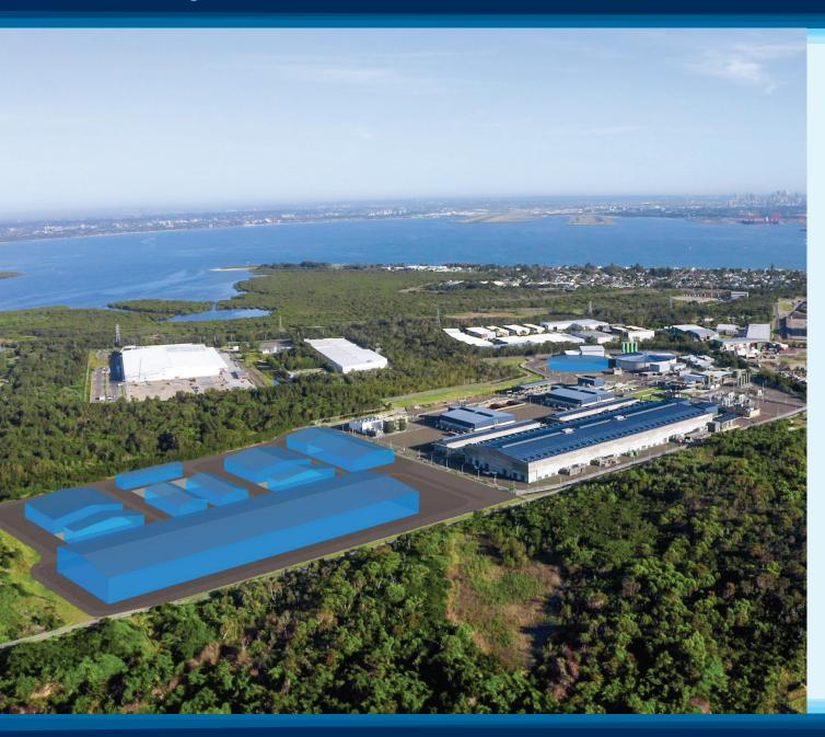
The Sydney Desalination Plant was originally constructed with expansion in mind, with the expectation that in the future it could produce up to 500 million litres of high-quality drinking water a day – double its current capacity.
